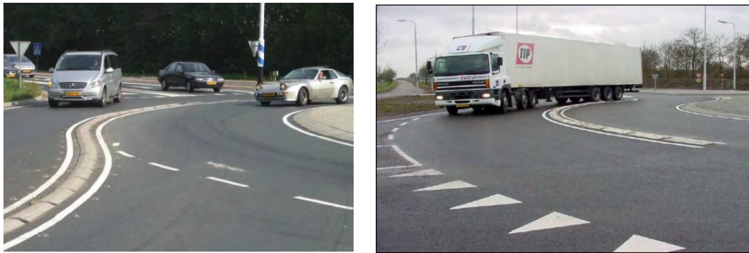
Figure 3. Turbo Roundabout Raised Lane Divider (Fortuijn)
